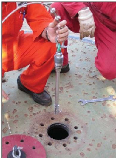
Application of corrosion coupons
